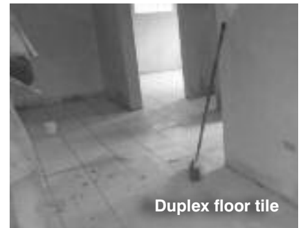
Duplex nearing completion
