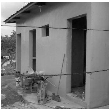
New bathrooms exterior
