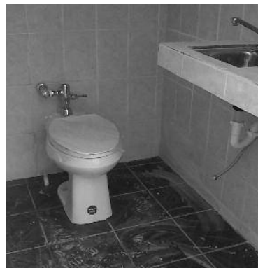
New bathrooms interior
